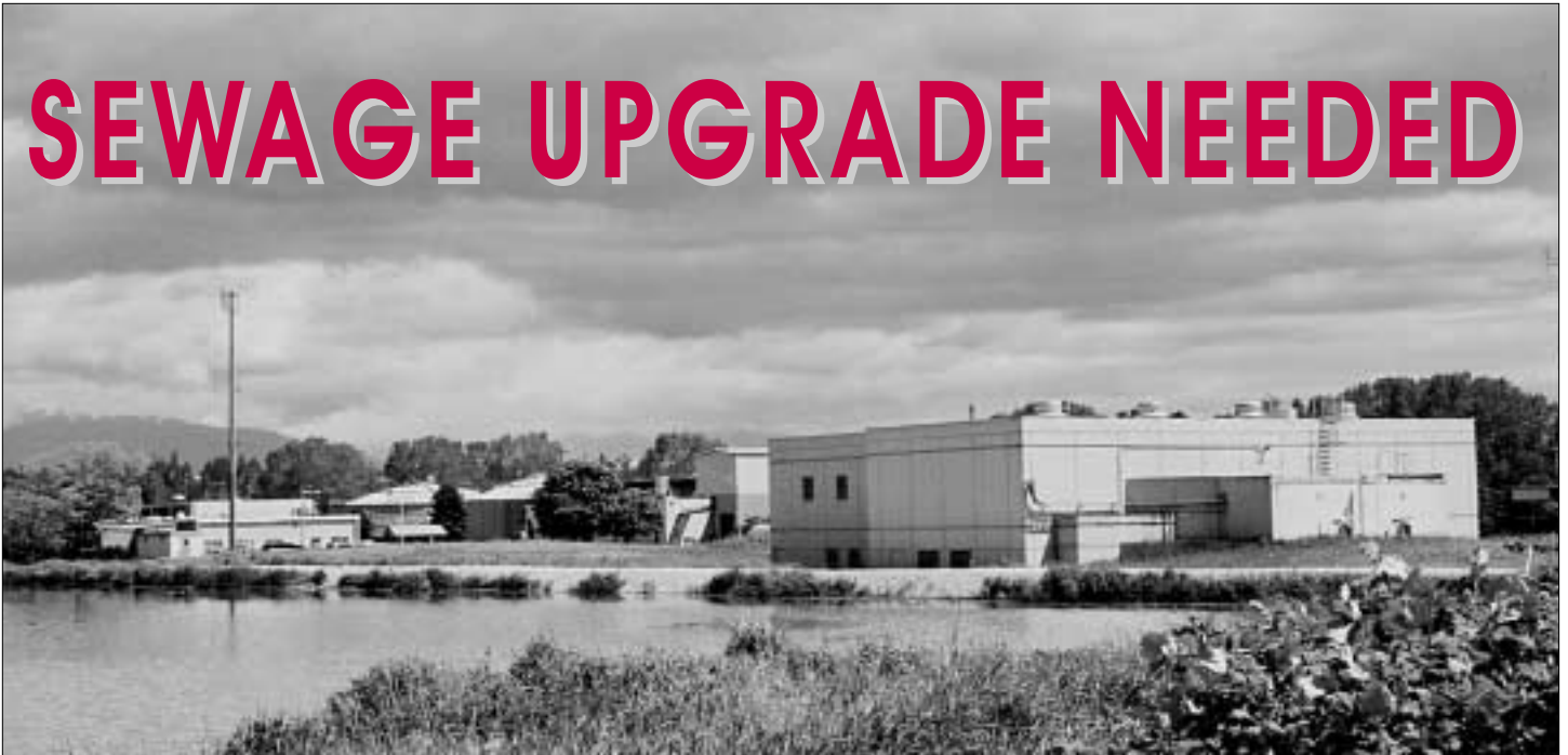
Iona Sewage Plant on Sea Island provides only minimal sewage treatment.
